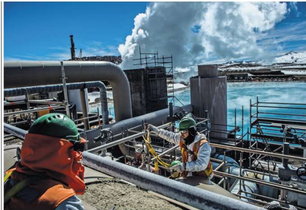
Workers installing pipe insulation at South America's first geothermal energy plant, located in Cerro Pabellón, Chile. The new plant will be able to power about 165,000 homes.
